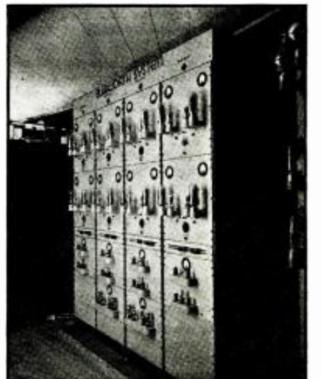
A portion of the amplifying equipment used in the super-power, 3-dimension sound system at the Lagoon of Nations, New York World's Fair, 1939. Frequency range: 28 to 11,000 cycles!
